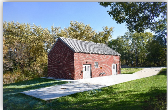
Example – South Milwaukee Lift Station
