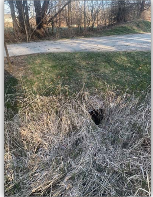
Arch culvert beneath drive
