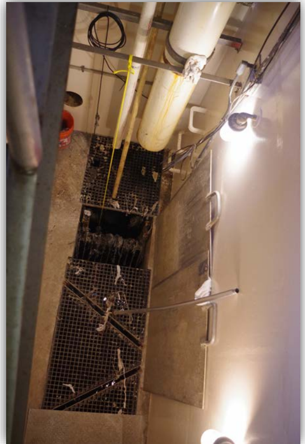
Influent wet well channel
