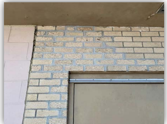
West expansion joint
