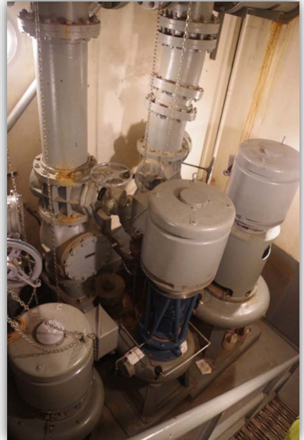
Corrosion of the concrete structure
