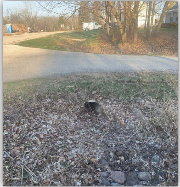
15-inch culvert beneath the station drive
