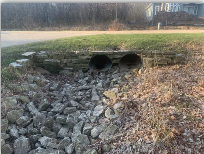
Two arch culverts beneath W. Ranch Road
