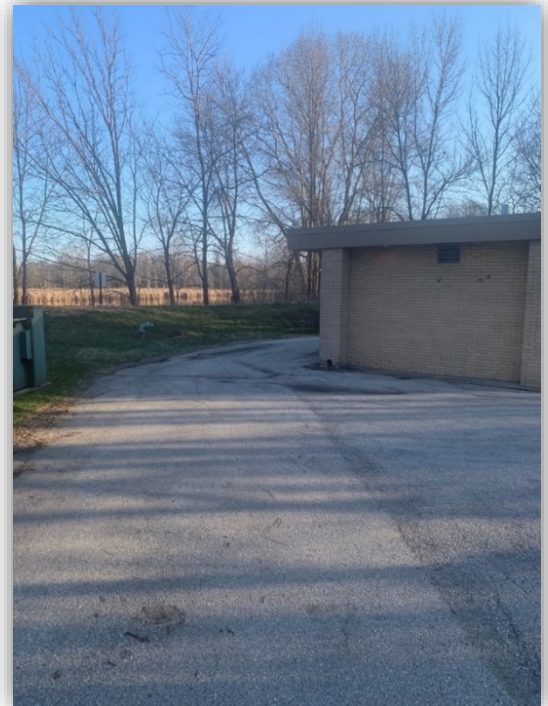
Berm on west side of station
